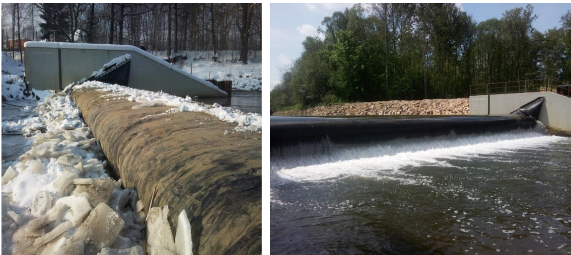
Figure 67: Inflatable weir in winter and summer seasons, Kliczkow SHP - Kwisá river, Poland (Polniak, 2015)
