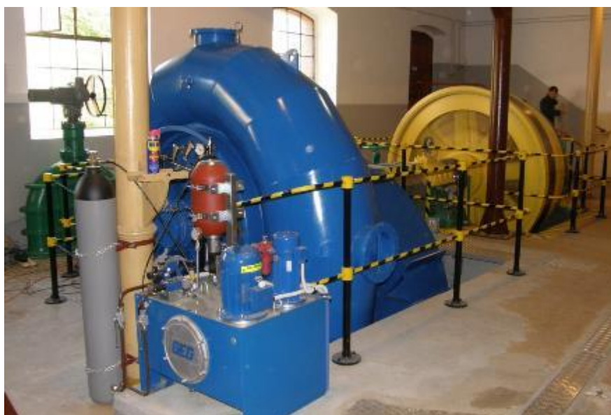
Figure 20: A modern Francis turbine in a refurbished Polish hydropower plant (source: IMP PAN archives)
