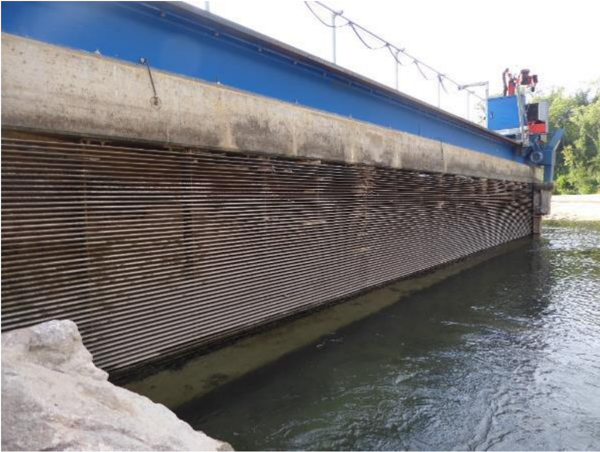
Figure 88: The horizontal bar rack of residual flow HPP Schiffmühle, Switzerland, during reservoir drawdown in July 2018 (source: J. Meister, VAW)
