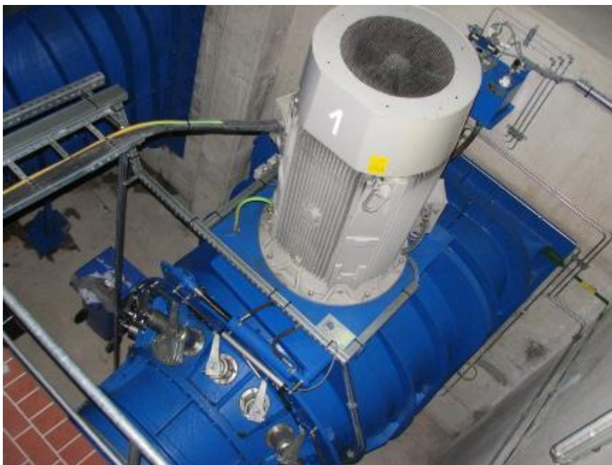
Figure 30: A typical compact unit with bevel speed increaser. Oborniki SHP, Poland (source: IMP PAN archives)
