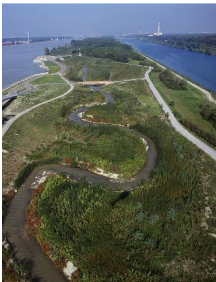
Figure 78: Nature like fishway at Freudenau HPP, Austria (source: W. Reckendorfer)
